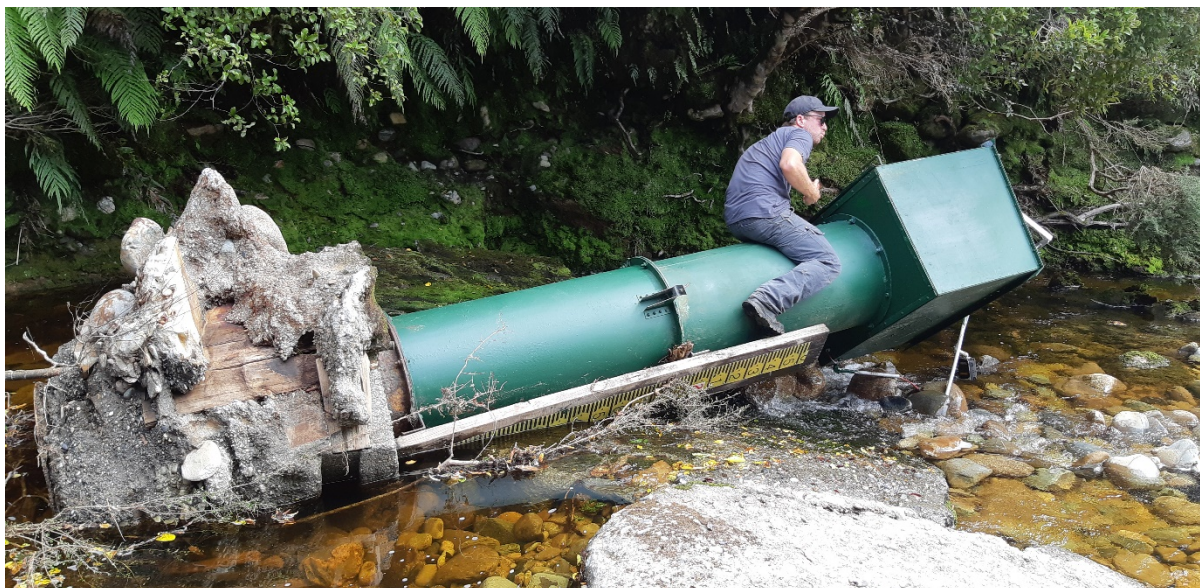
Figure 1: Flood damage to the Butchers Creek flow recorder after the 4 February 2020 floods.
